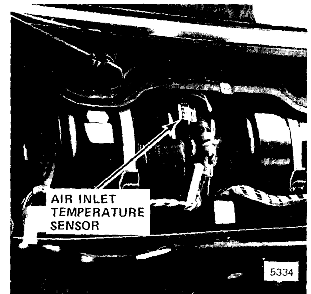
Figure 5 - Under Center Of Fresh Air Intake Cowl
