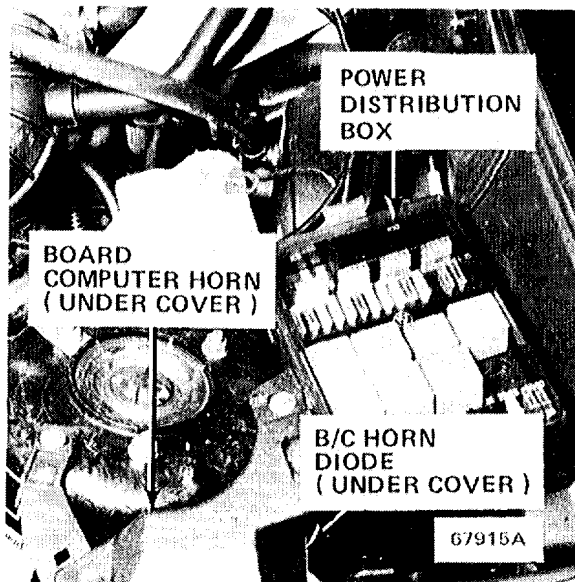
Figure 1 - LH Rear of Engine Compartment
